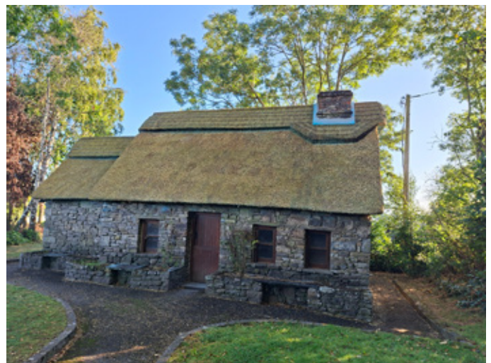
Final thatched roof
